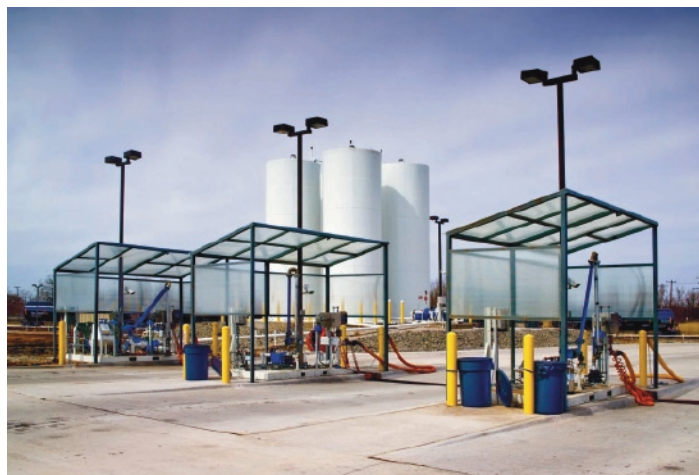
Oklahoma city terminal – completed June 2008
